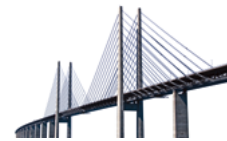
BRIDGES more weatherproof
